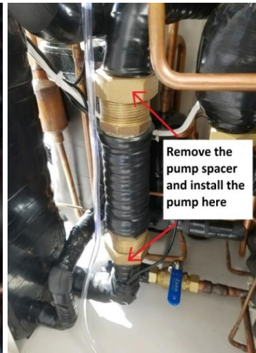
Removing the shipping spacer
