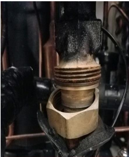
Peel back the insulation
